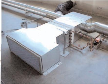
placed right up to the wall while allowing air to be discharged at the base of the window. One UFT supplies up to six linear grilles designed to handle a maximum of 210 cfm each.
