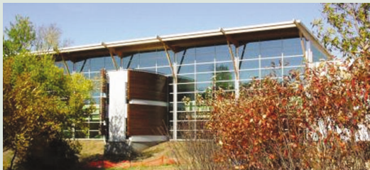
Johnson County Sunset Drive Office Building, Olathe, Kansas; Designed to LEED Gold
